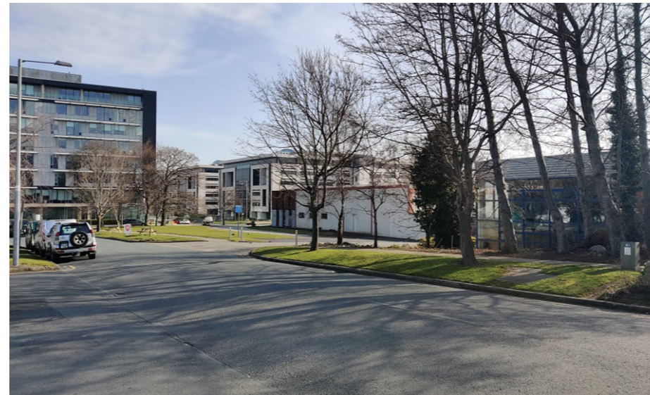
View looking North from Ravens Rock Road (Site to Right)
