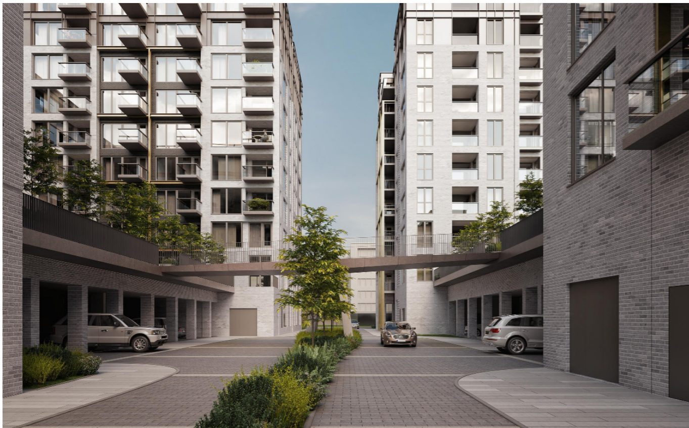
NEW INNER ROAD - VIEW TOWARDS CARMANHALL ROAD
